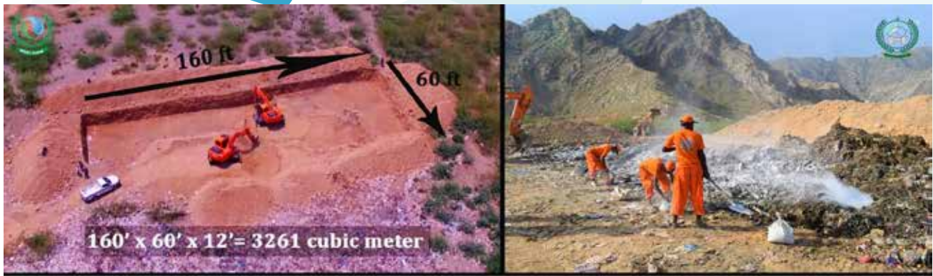
Aerial view of Pit excavated for safe disposal of animal waste during Eid Ul Azha by WSSCK
