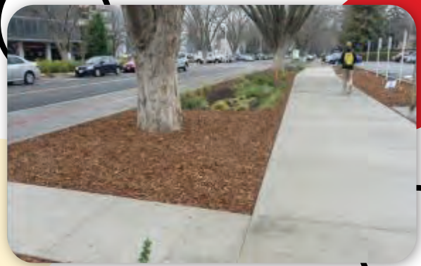
Green Streets with Infiltration swales
