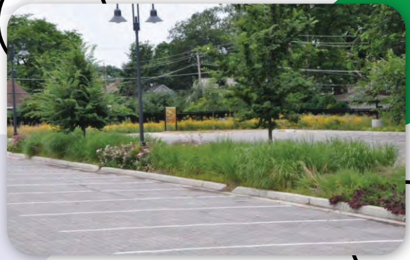
Permeable paving Drains used in to vegetated swale used in Parking lot, Elmhurst, Illinois, USA
