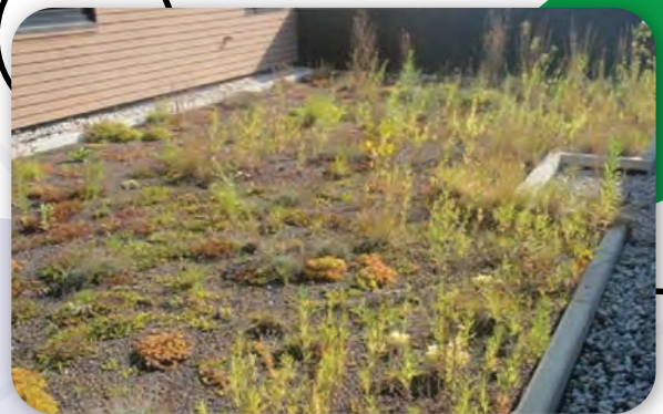
Green Roof in Villa Park, Illinois, USA
