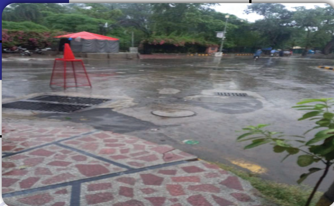
Fig 19: View of Lawerence Road after the construction of Stormwater Storage Tank
